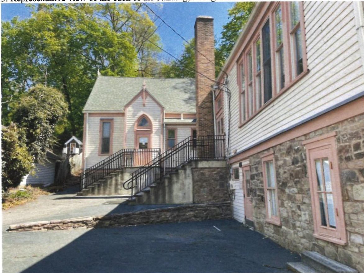
4. Representative view of the western side of the building, facing north.
