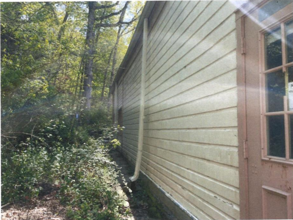
5. Representative view of the back of the building, facing east.
