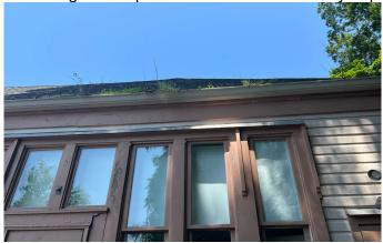
8) The rear of the building has a facing slope that could lead to water damage during a storm – rainwater runoff and gutter drainage should be examined by a qualified engineer:
